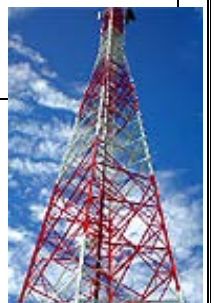
Cell phone transmission tower
